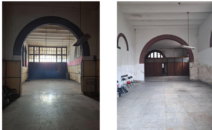
Figure 5. Daylight barrier panels to the interior
