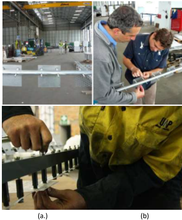
Figure 4. ( a) Aluminium Panel Construction and (b) Assembling Process
