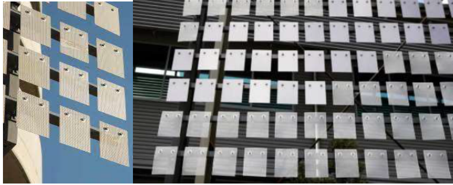
Figure 3. Kinetic Facade Panels at Brisbane Airport
