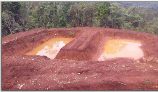
Gambar 9: Settling pond PT. XYZ model zig-zag
