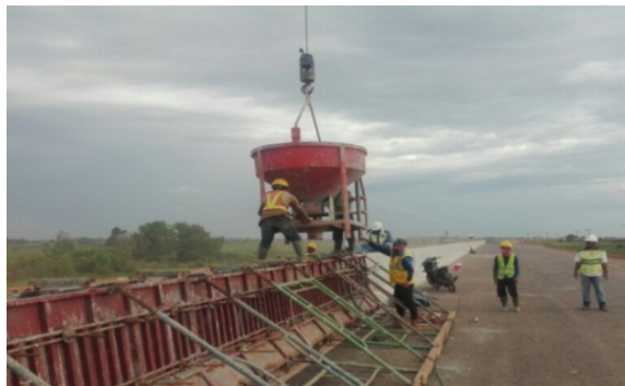
Figure 1. Concrete Barrier Making with Manual Formwork
