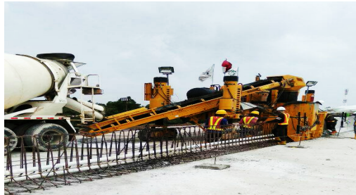
Figure 2. Making Concrete Barrier with Slipform Paver
