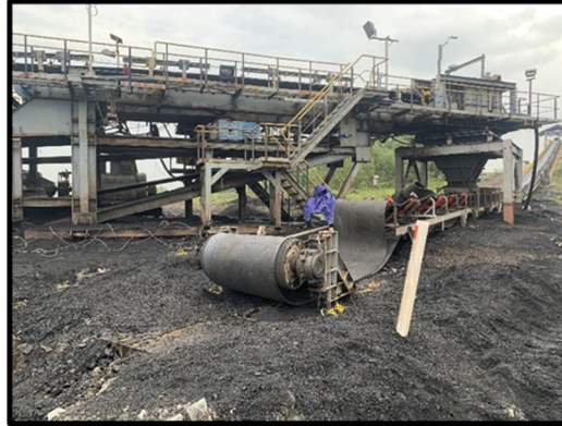
Gambar 3. Pengantian sabuk ban Belt Conveyor
