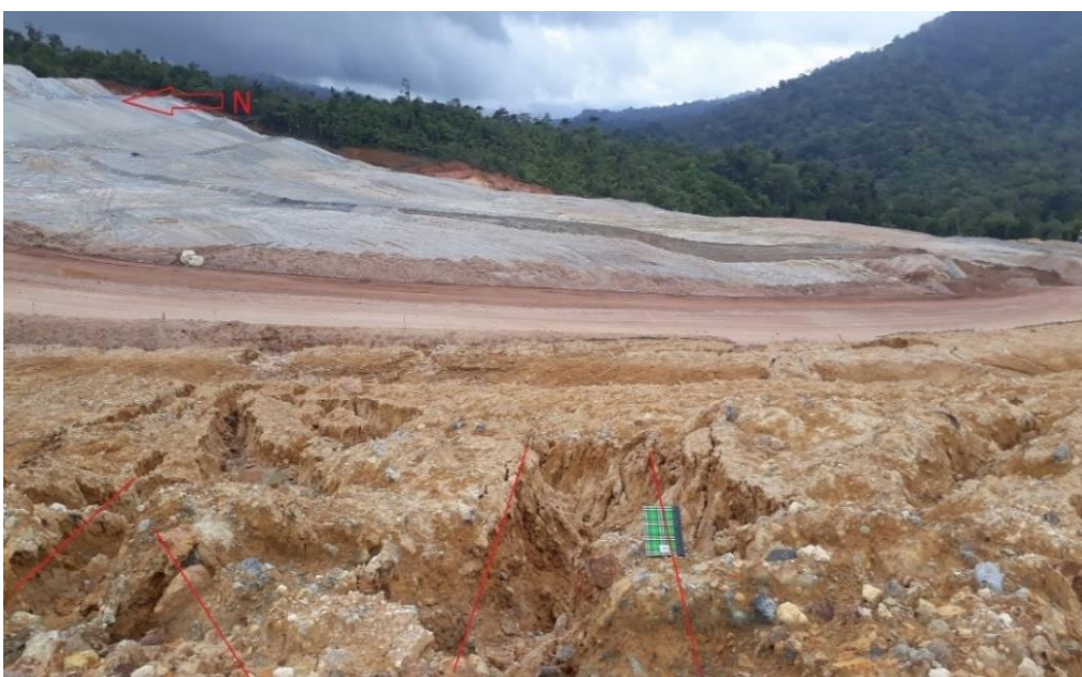
Figure 12. Conditions scraping in waste dump 1c
