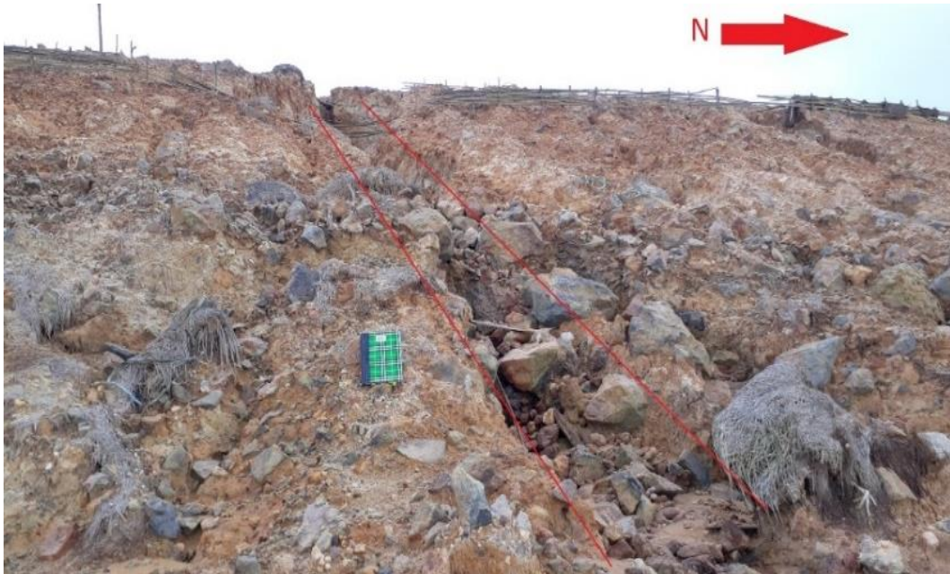
Figure 5. Field condition of water runoff flow in waste dump 1a
