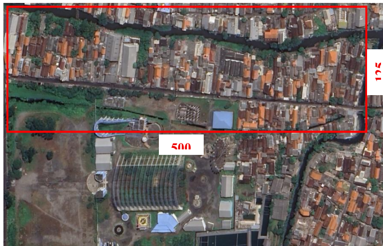
Figure 1. Study area along Kolonel Sugiono Street (Source: Google Maps)
