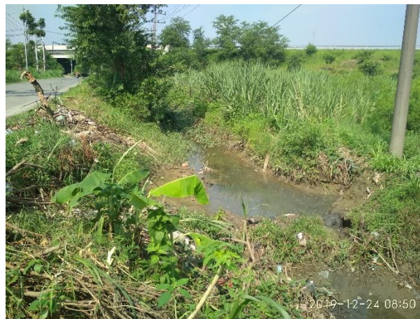
Figure 3. Drainage Channel's Existing Condition
