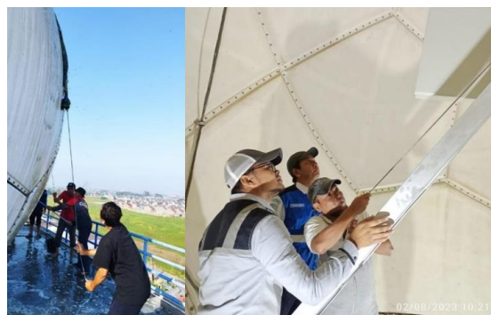
Fig. 2 Weather Radar Maintenance
