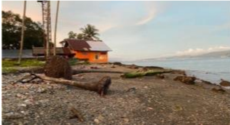
Figure 5. Beach Abrasion Condition (November 23, 2022)
