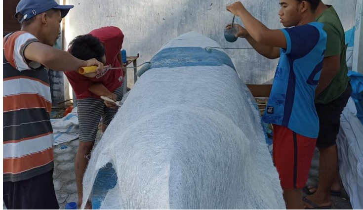
Gambar 5. Pelapisan Fiberglass Reinforced Plastic (FRP)
