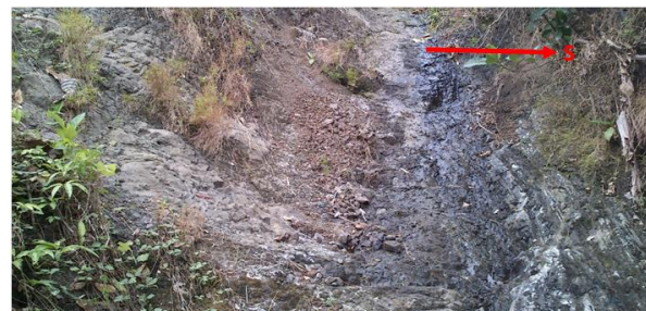
Figure 16. Photo of the location of data collection for the JN 40 shear fracture.
